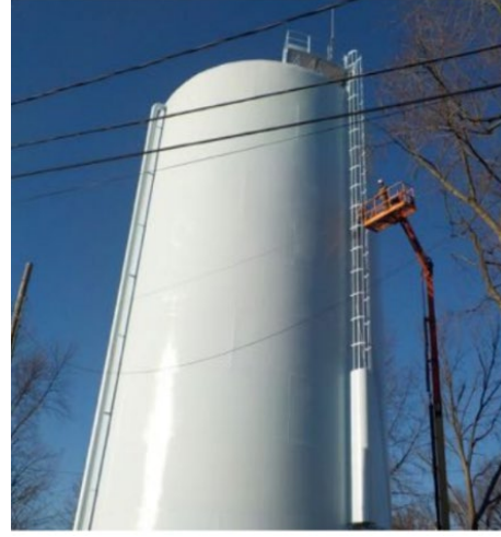
High Street tank exterior before and after blasting and painting.
