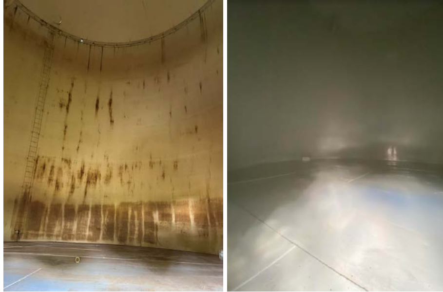
Turnpike tank interior before and after interior blasting and painting.
