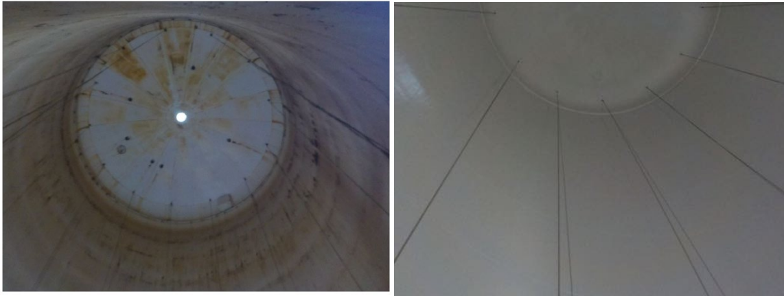
High Street tank interior before and after interior blasting and painting.
