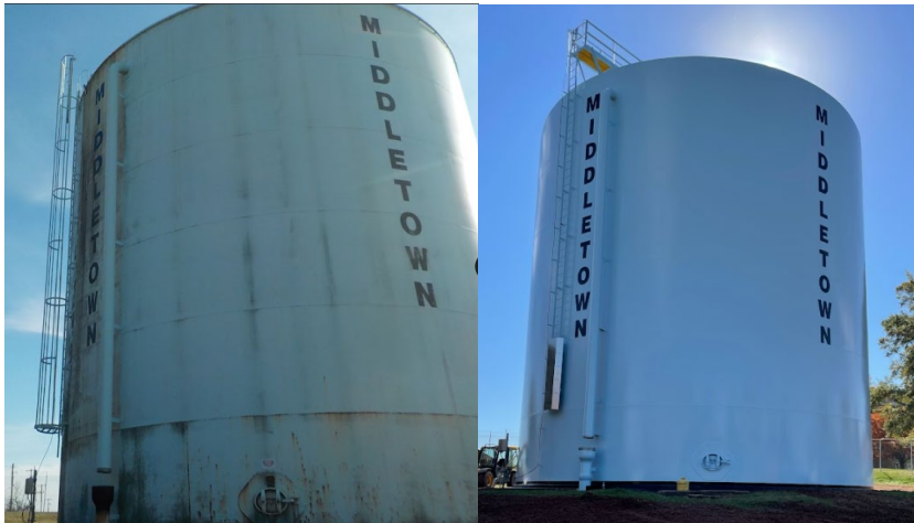
Turnpike tank exterior before and after exterior blasting and painting.
