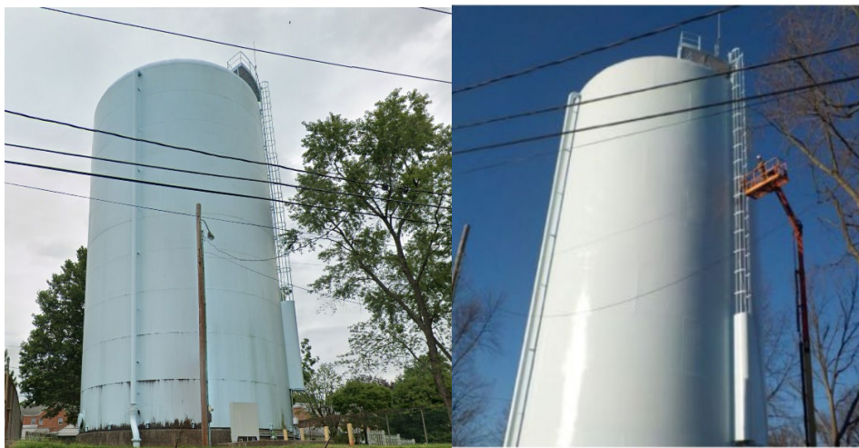
High Street tank exterior before and after blasting and painting.
