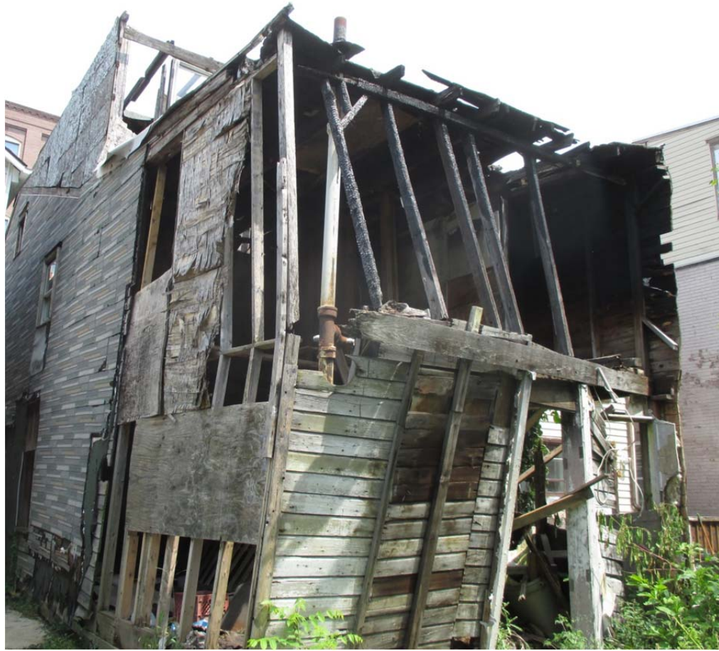
Photo No. 3: Rear of the house.
