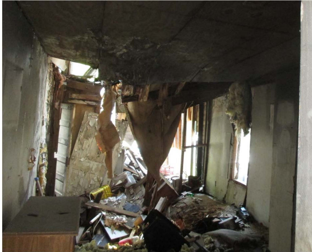
Photo No. 1: View of the first floor from the front door.
